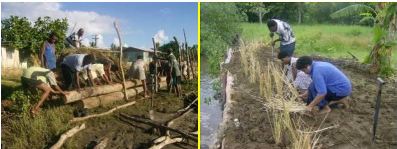
*Construction of river bank protection structures using local materials, and planting of vetiver grass for bank stabilization (Buretu, Fiji – USP CBA project)*
